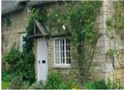
4.9 Many of the early 18<sup>th</sup> century thatch roofed cottages in the village typically feature windows with thin wooden lintels and small-paned timber glazed side-hung casements such as at no. 11 Deene End (see below) that has a thin central vertical glazing bar dividing the window into 8-panes.
