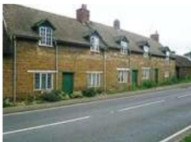
4.8 Many of the older cottages fronting Main Street still feature leaded-light windows set in wooden frames with wooden casements, such as nos. 2, 3, and 4 (see below). Originally this row was thatched, but this caught fire and the upper section of wall shows signs of rebuilding, the eaves dormers dating from the mid-20<sup>th</sup> century using a small-paned casement style.
