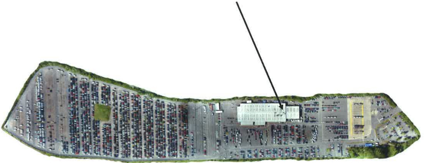
Location of extract ducts
